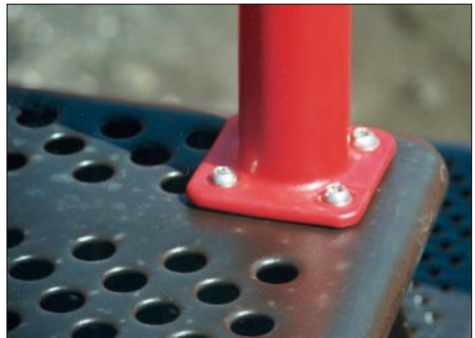
The products produced on the 1524 CNC are plates used to bolt play events onto the decks of the playground structures. These mounting plates keep the whole structure together.
