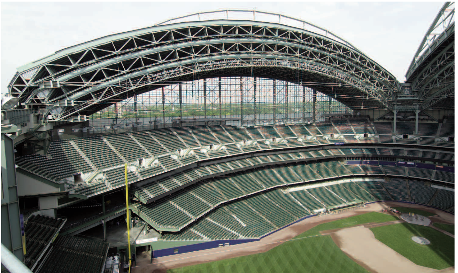
Miller Park Baseball Stadium's seven panel radial retractable roof.
